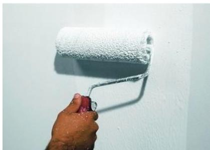
Step 1 - Start applying a first coat of Primus Sabbia with a brush on properly cleaned and insulated ceilings and walls.
