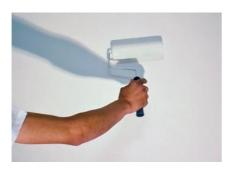
Step 3 - On the ceiling, apply the product with a medium-haired roller (if necessary, apply a second coat)
