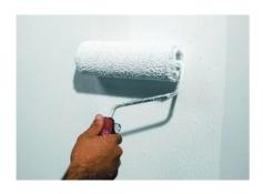
Step 1 - Start applying a first coat of Primus Sabbia with a brush on properly cleaned and insulated ceilings and walls.
